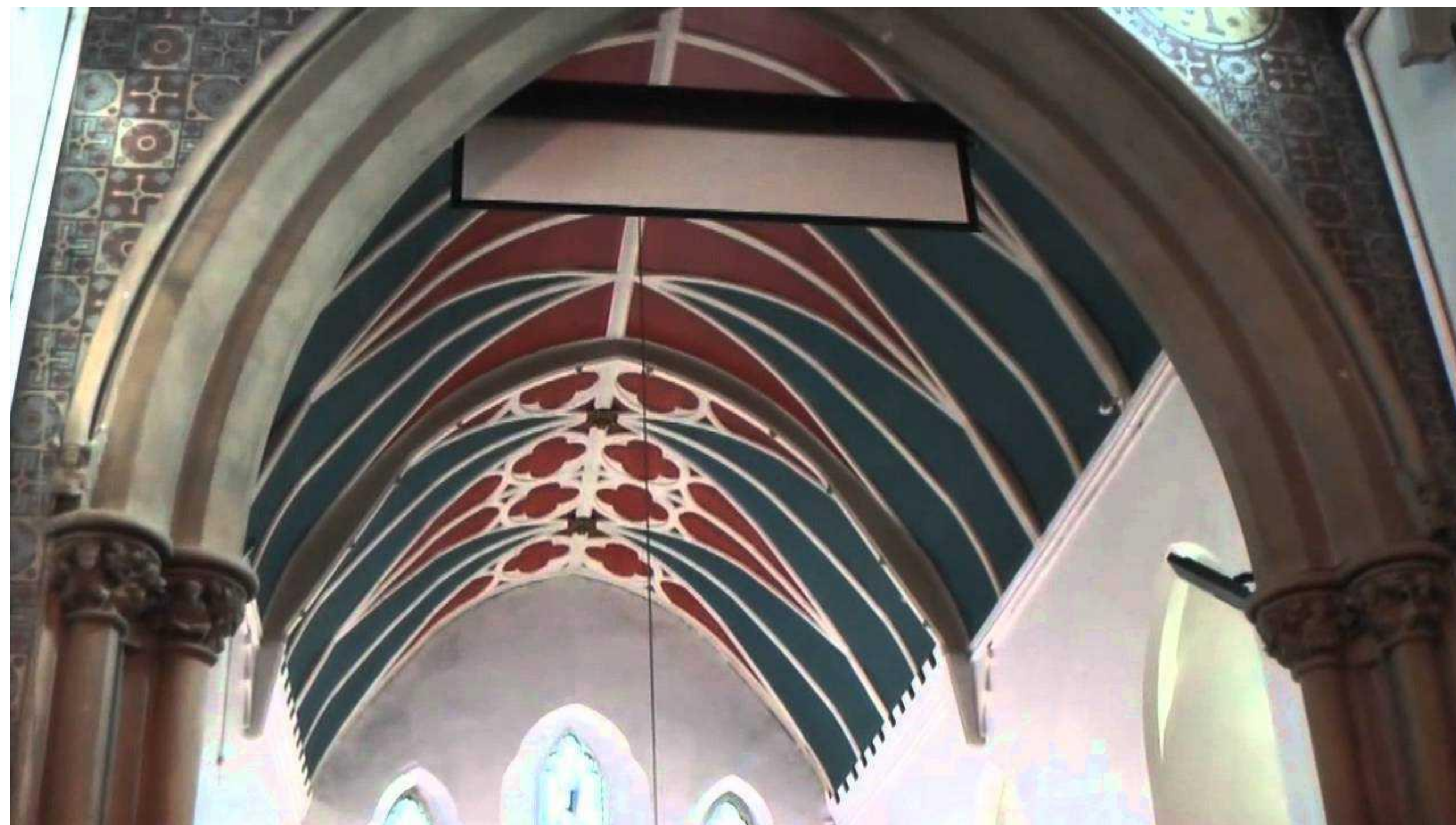
View in front of arch showing screen winch system starting to lower and screen material beginning to roll out
