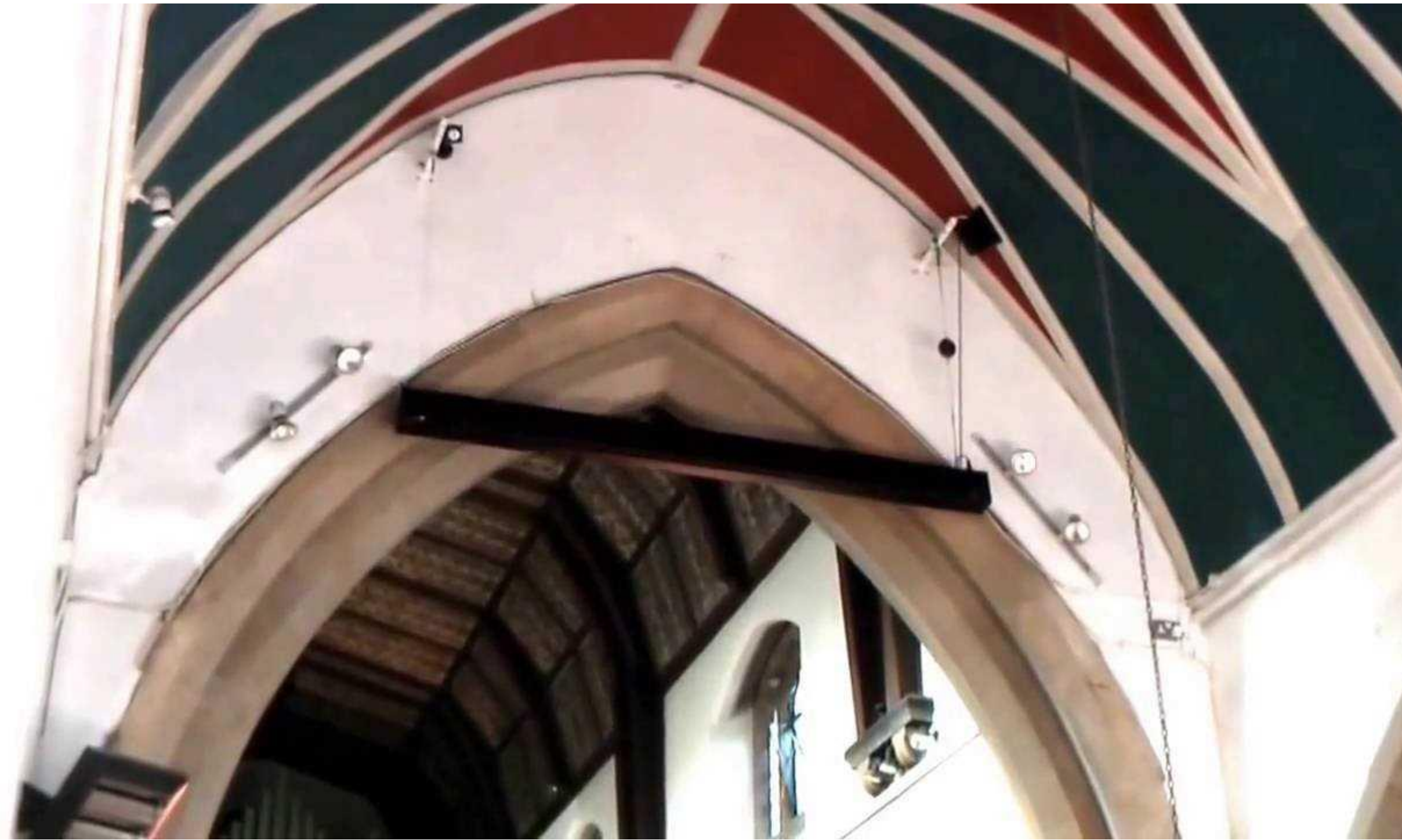
View behind arch showing screen winch system starting to lower, prior to screen material rolling out
